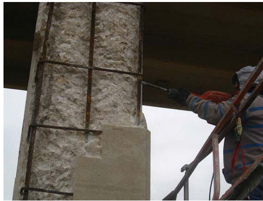
Figure 3-3. Chipping hammer used to remove unsound concrete.
