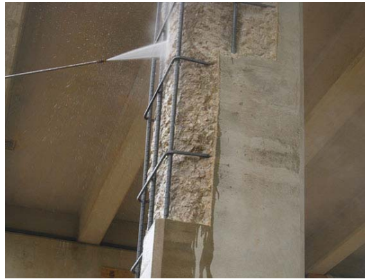
Figure 3-7. Pressurized water to clean and prepare surface (saturated surface dry).
