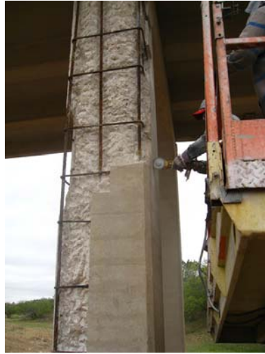
Figure 3-2. Preparation (saw-cutting) straight and squared edges to contain patch material.
