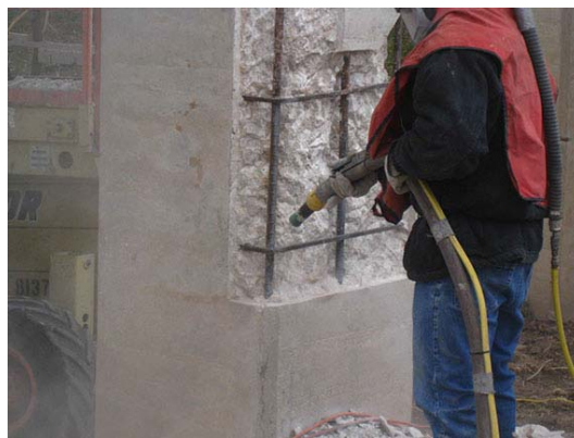
Figure 3-5. Abrasive blasting to clean reinforcing of rust/active corrosion.
