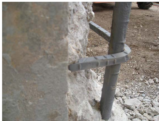
Figure 3-6. Reinforcing cleaned and free of rust.
