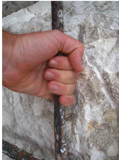
Figure 3-4. Verifying adequate clearance around reinforcing.
