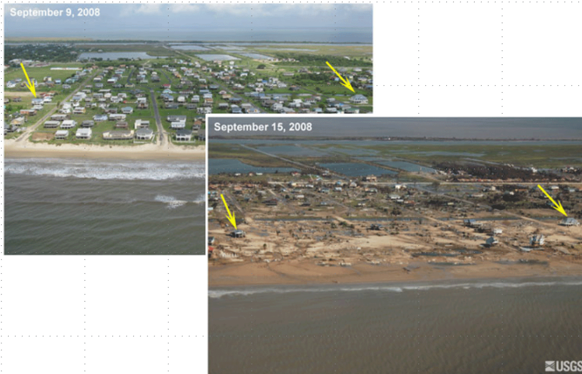
Figure 15-17. Damages on Bolivar Peninsula following Hurricane Ike.
