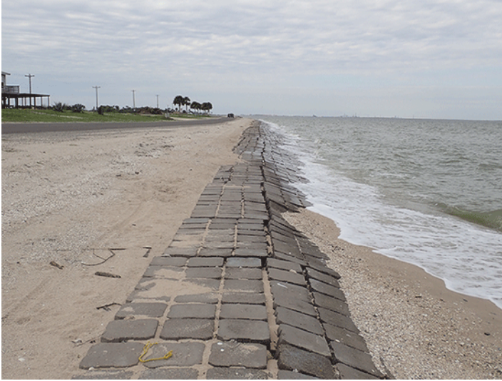
Figure 15-27. Cellular Concrete Mattresses Protecting a Coastal Highway in Calhoun County, Texas.
