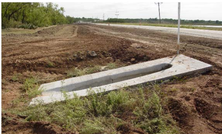
Figure 8-3. Pipe mitered to conform to fill slope.
