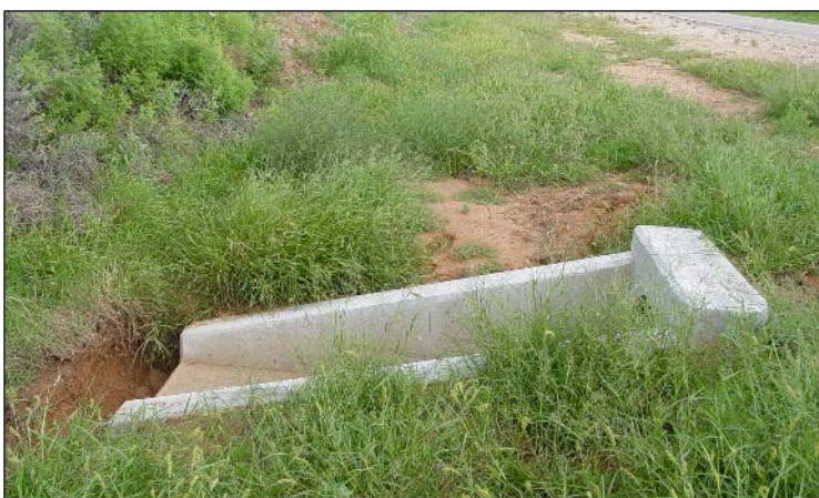
Figure 8-5. End section conforming to fill slope
