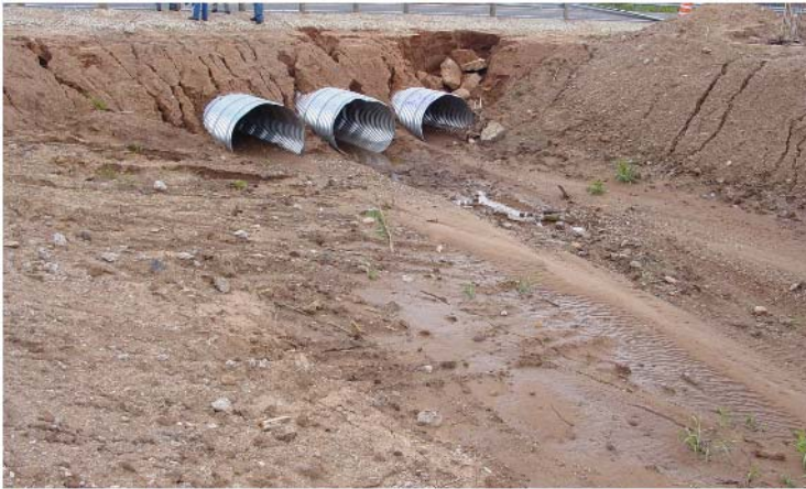
Figure 8-31. Temporary or Detour Culverts
