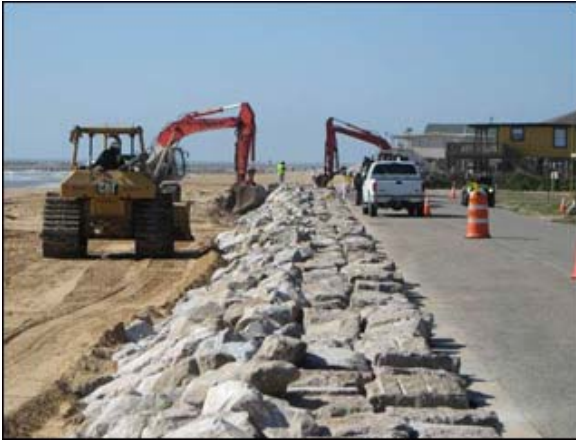
A - Revetment construction along CR257 in Brazoria County, Texas (Apollo Environmental)
