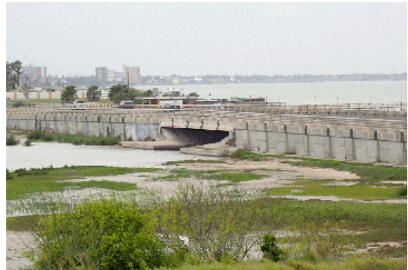
D - Vertical walls provide roadway protection along this Ocean Drive crossing in Corpus Christi, Texas
