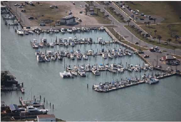
C - Bulkheads protecting roadways in Aransas County, Texas
