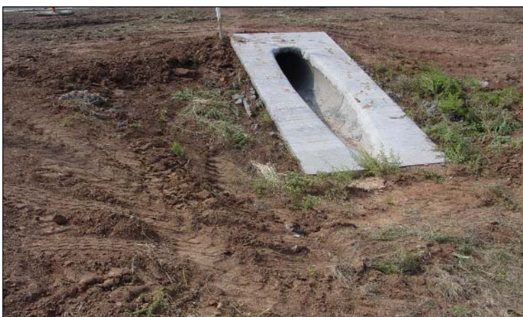
Figure 8-4. Pipe mitered to conform to fill slope.
