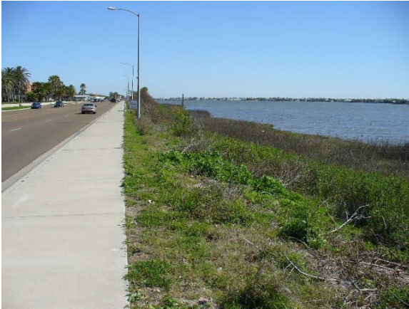
A - Wetlands and submerged oyster reef barriers provide living shoreline protection for Broadway Street in Aransas County, Texas
