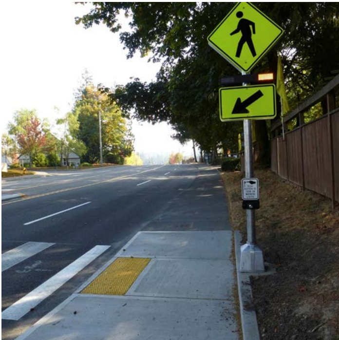
Figure 7-33. Rectangular Rapid Flashing Beacon.
