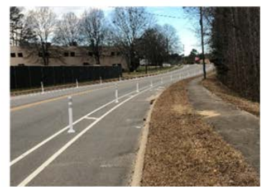
Raleigh, NC. Street Level with Flexible Post Separation
