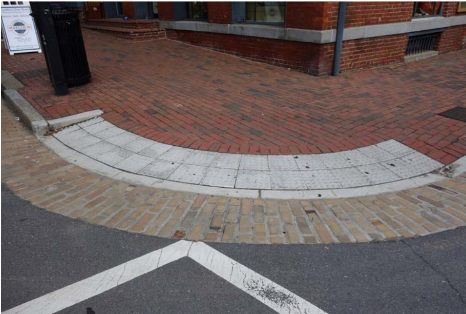
Figure 7-14. A Blended Transition Curb Ramp.
