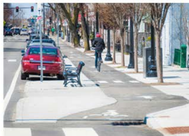
Cambridge, MA. Sidewalk Level with Parking Separation
