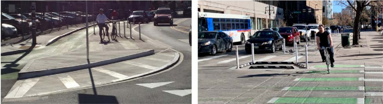
Figure 6-46. Protected Corner Treatment Details: Truck Apron (left) and Turning Wedge (right)
