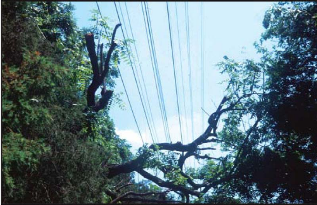
Figure 4-22. Unacceptable pruning by utility. Limb stubs left unpruned.
