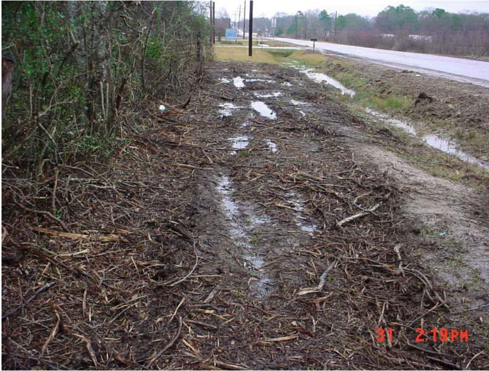
Figure 4-24. Pruning debris not removed and right of way damage by utility.
