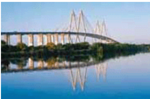
Figure 11-11. Fred Hartman Bridge over the ship channel.
