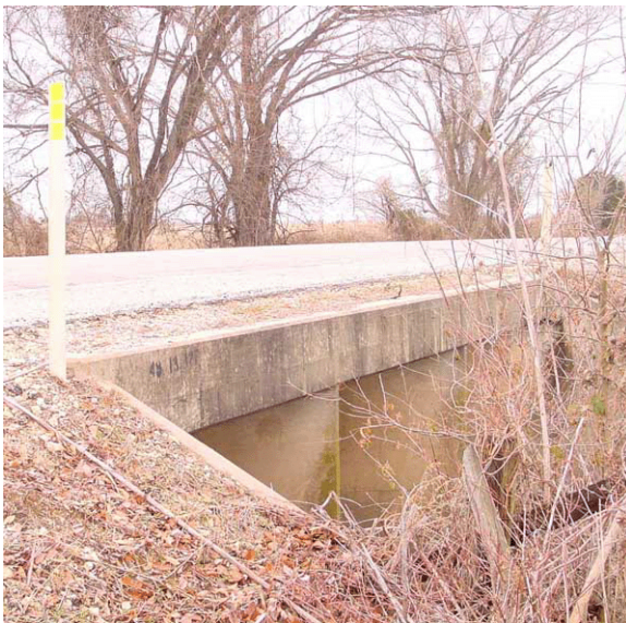
Figure 11-22. Multiple box culvert.
