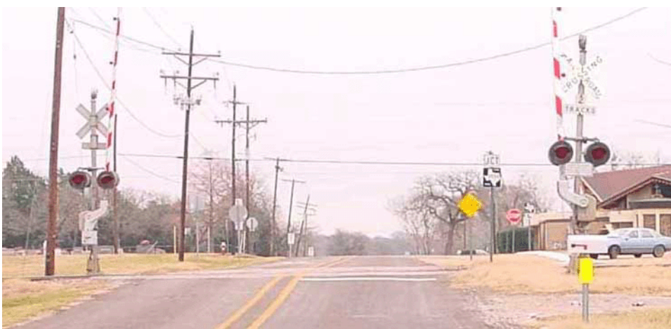
Figure 11-9. At-grade railroad crossing.
