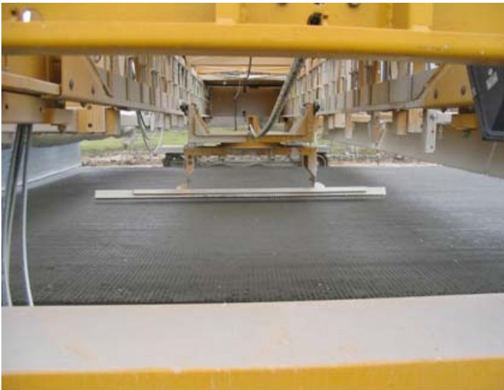
Figure 9-62. Mechanical tining device.
