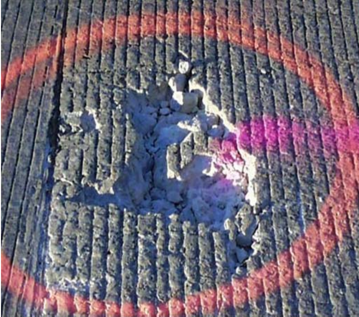
Figure 10-2. Deep spalling.
