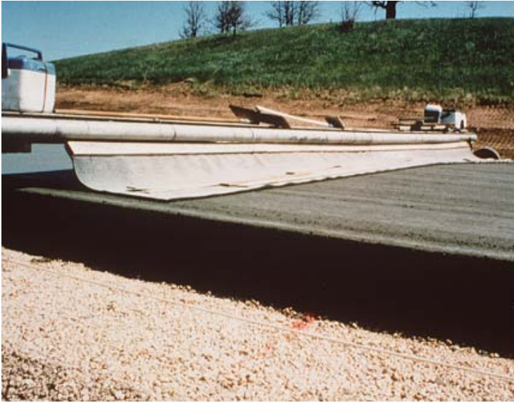
Figure 9-59. Artificial carpet drag.
