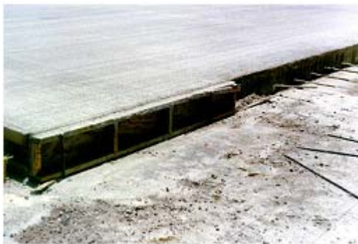
Figure 9-78. Wood side form at a transverse construction joint.
