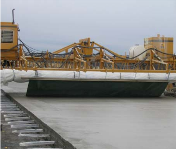
Figure 9-60. Mounting of artificial carpet.
