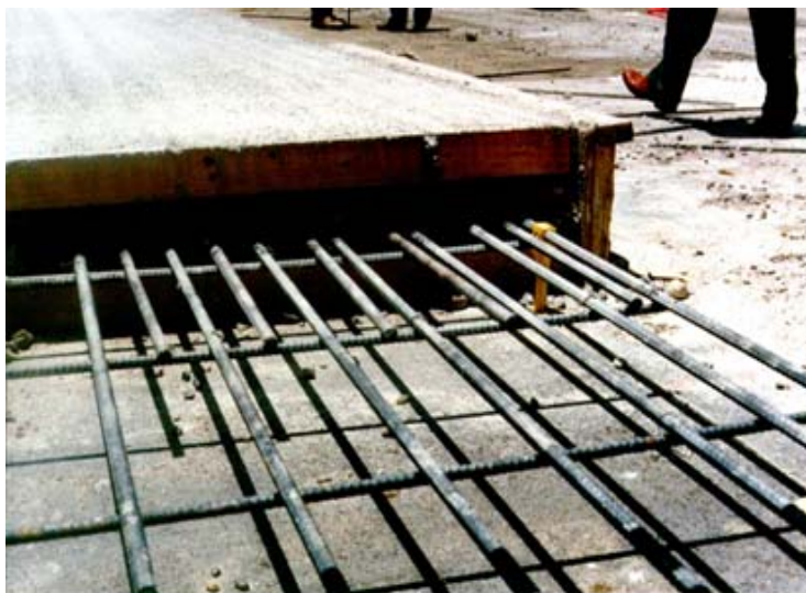
Figure 9-76. Additional steel is required at header.
