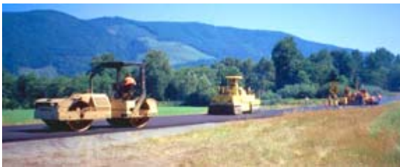
Figure 6-60. Breakdown and Intermediate Rollers. © Copyright 2006 University of Washington
