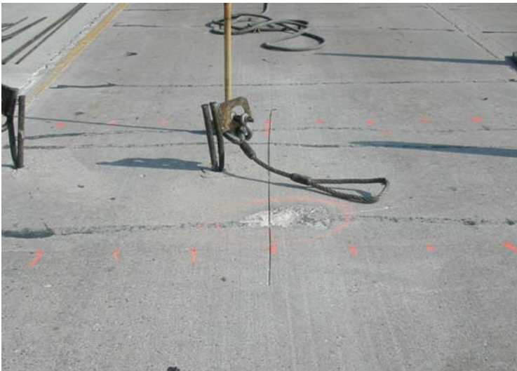
Figure 10-4. Slab ready for lifting.
