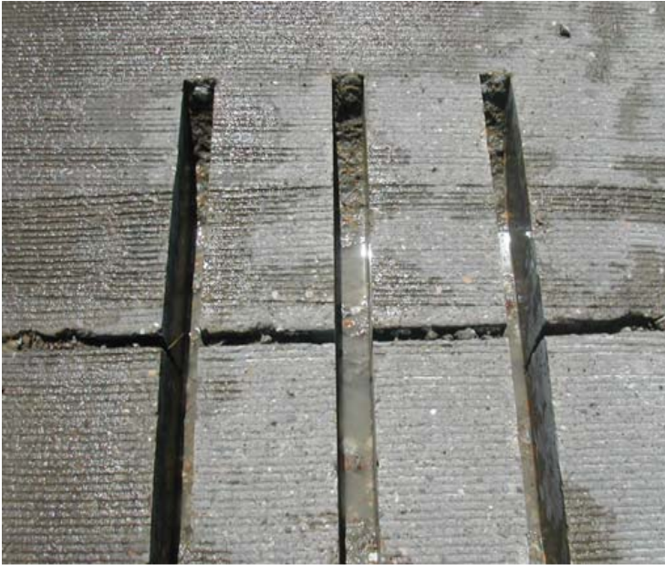
Figure 10-22. Flat bottom after being water cleaned.
