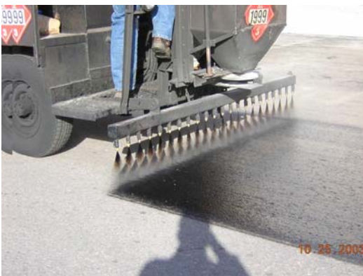
Figure 6-10. Tack coat application showing nozzle coverage area. © Copyright 2006 University of Washington
