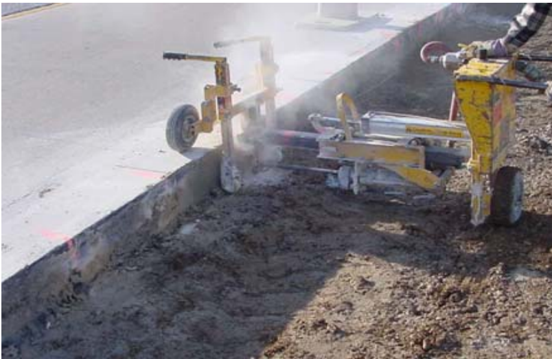
Figure 9-80. Marking and drilling holes at widening joint.
