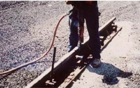
Figure 9-22. Using jackhammer to set staking pin.
