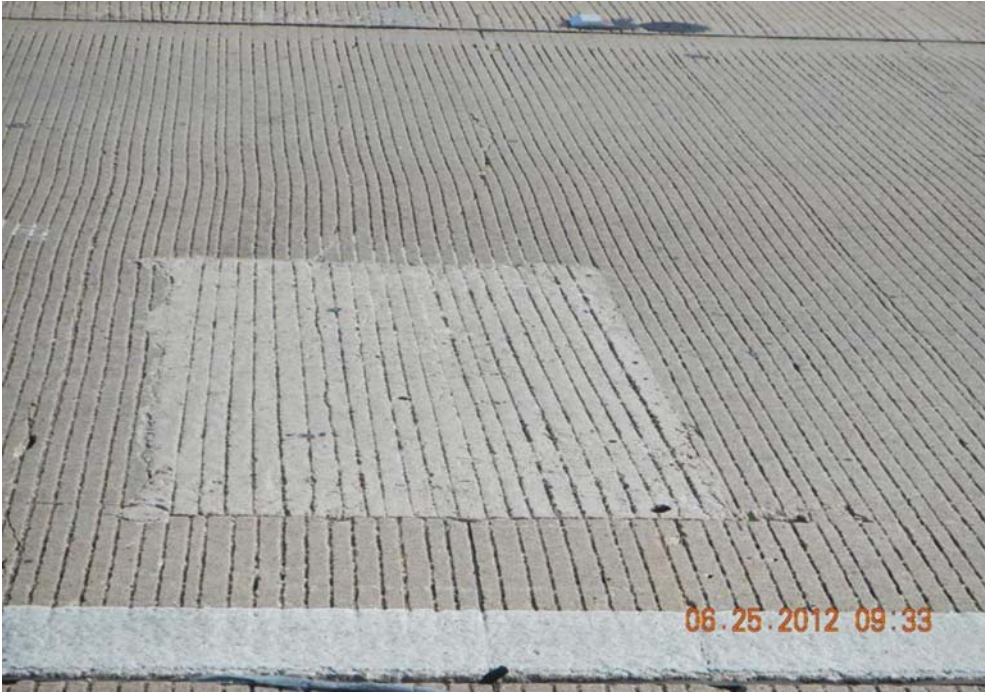
Figure 10-13. Finish the surface.
