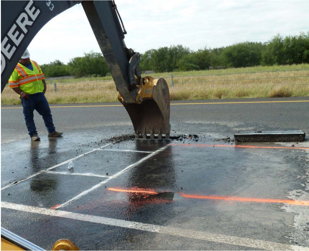
Figure 4-19. Removing hot-mix asphalt (HMA) block with backhoe.
