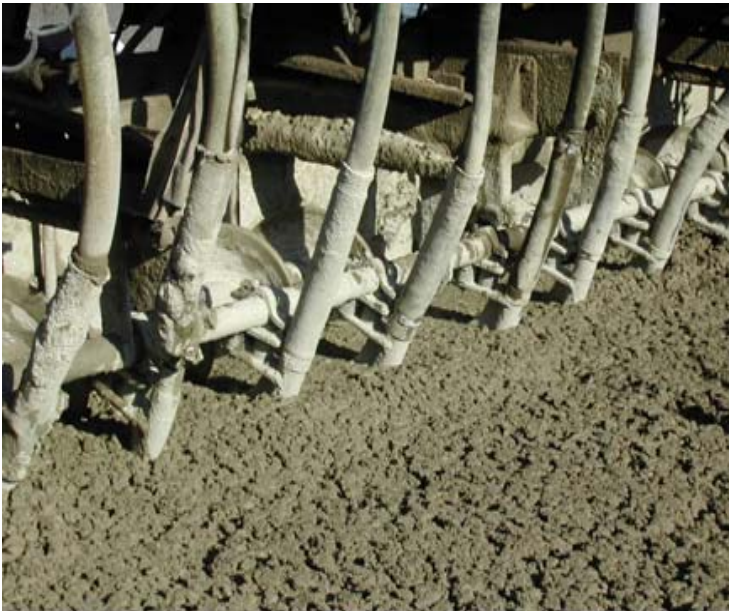
Figure 9-44. Immersion vibrators.
