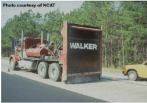
Figure 7-5. Drop hammer “breaking” slab for “break and seat.” © Copyright 2006 University of Washington
