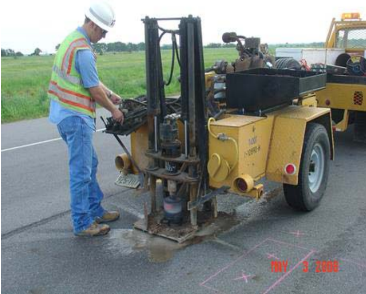
Figure 4-21. Coring using a water-cooled barrel.
