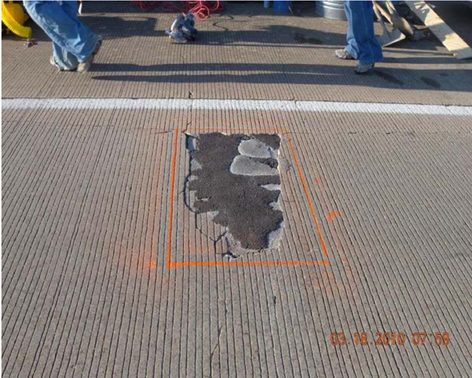
Figure 10-8. Identify the repair limits.
