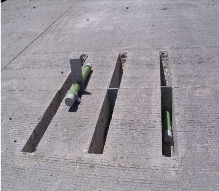
Figure 10-23. Dowel bar in place for backfill material application.
