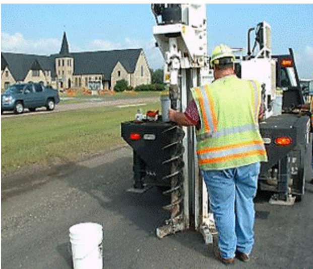
Figure 4-23. Augering a pavement for material samples.
