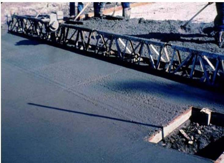
Figure 9-26. Vibrating screed.
