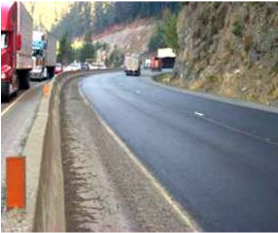
Figure 6-32. Gearbox streak in a new mat. © Copyright 2006 University of Washington
