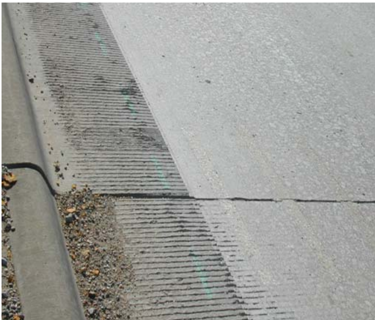
Figure 10-24. After DBR, slab jacking, and diamond grinding of the section shown in Figure 10-17.
