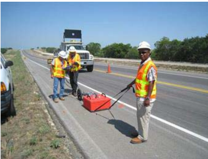
Figure 4-10. 200 MHz Ground-coupled Penetrating Radar.
