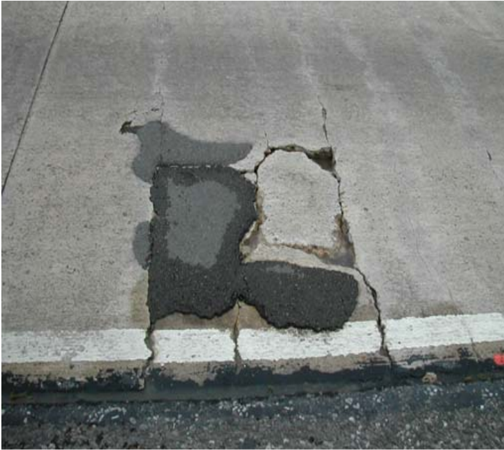
Figure 10-1. Typical punchout in CRCP.
