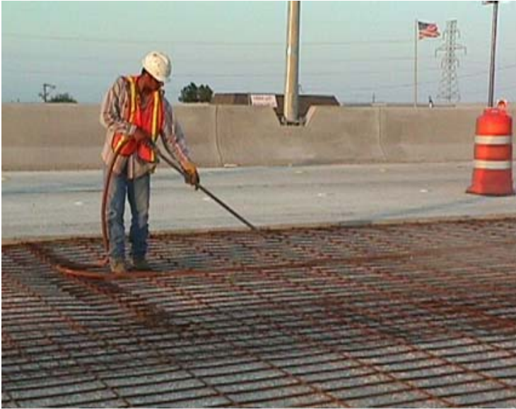
Figure 10-15. Airblasting to clean the concrete surface.
