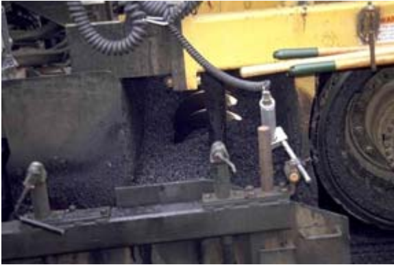
Figure 6-29. Augers distributing HMA. © Copyright 2006 University of Washington
