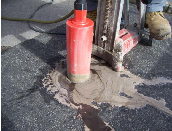
Figure 6-52. Core extraction. © Copyright 2006 University of Washington
