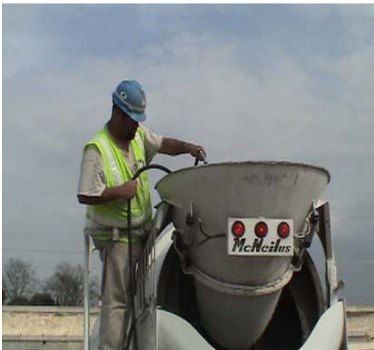
Figure 9-12. Washing the mixer drum.
