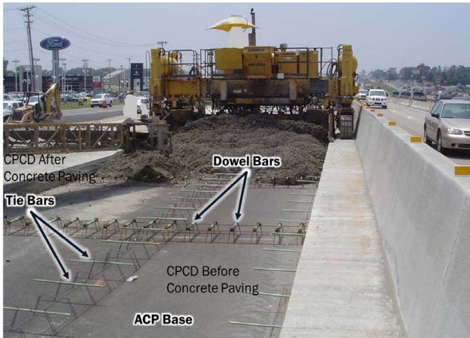
Figure 8-2. Concrete Pavement Contraction Design.
