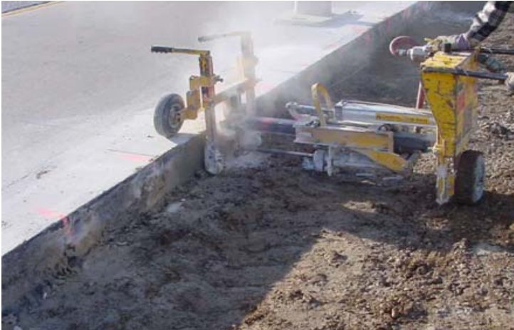
Figure 10-5. Drilling holes at longitudinal joint.
