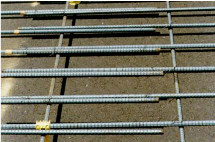
Figure 9-14. Spliced or lapped longitudinal steel.
