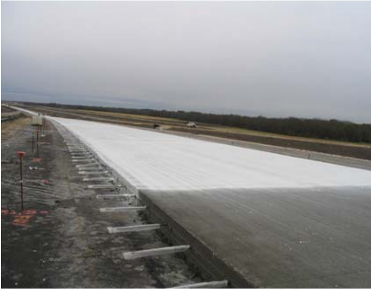
Figure 9-67. Preventing curing compounds from dropping on tie bars.
