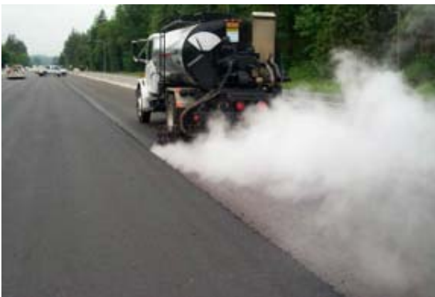
Figure 6-9. Tack coat application. © Copyright 2006 University of Washington
