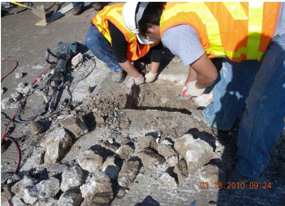
Figure 10-10. Removing deteriorated concrete.
