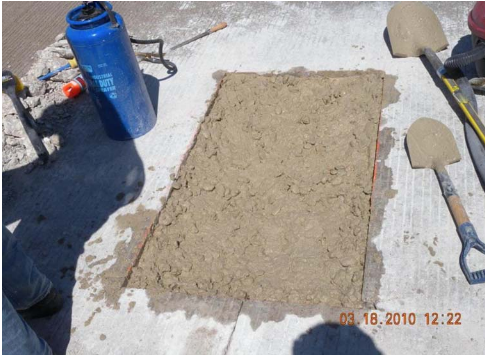
Figure 10-12. Place repair materials.
