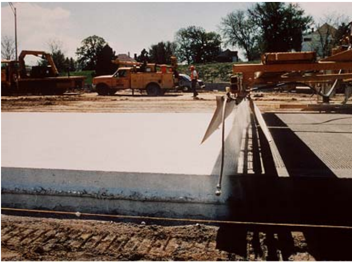
Figure 9-64. Mechanized spraying unit.
