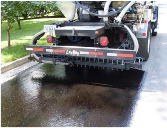
Figure 6-6. Tack Coat Distributor Truck Spray Bar. © Copyright 2006 University of Washington
