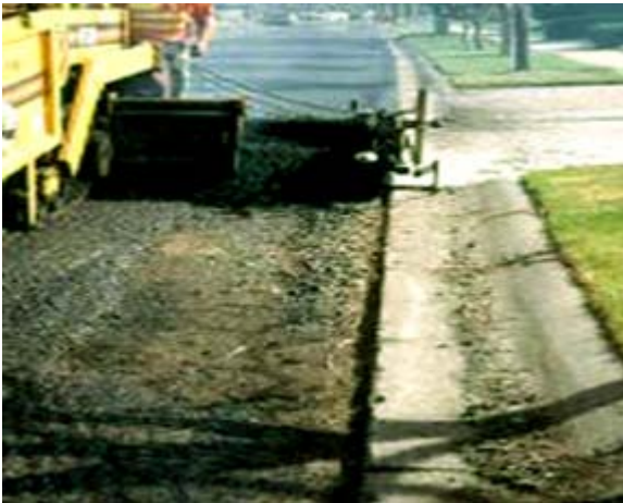
Figure 6-37. Screed Extension. © Copyright 2006 University of Washington
