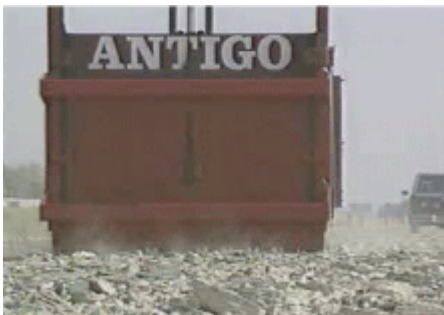
Figure 7-4. Drop hammer breaking slab for break and seat operations. © Copyright 2006 University of Washington
