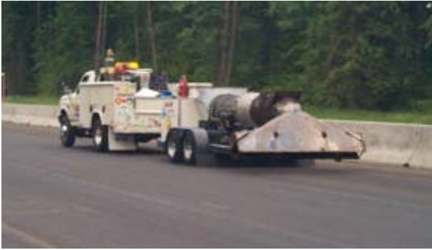
Figure 6-8. Jet dryer used ahead of the tack coat distributor. © Copyright 2006 University of Washington
