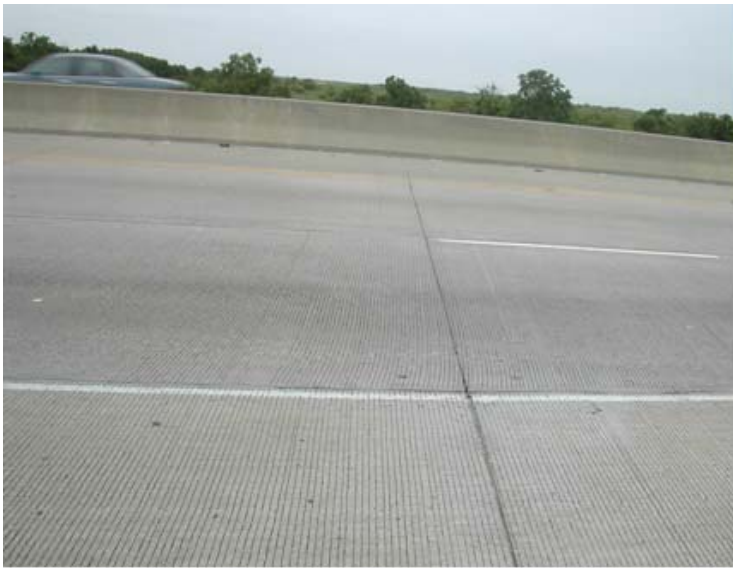
Figure 9-69. Transverse contraction joint.
