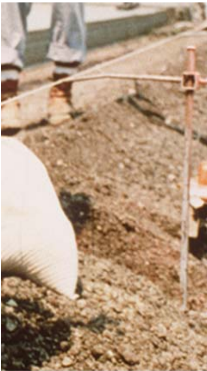
Figure 9-39. Guide wire controls.
