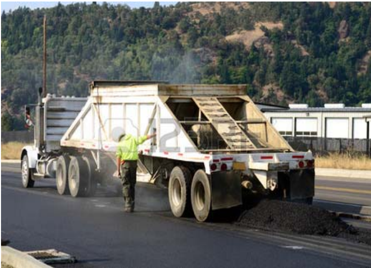
Figure 6-14. Bottom dump truck. © Copyright 2006 University of Washington
