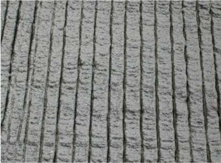
Figure 9-61. Transverse tined Surface.
