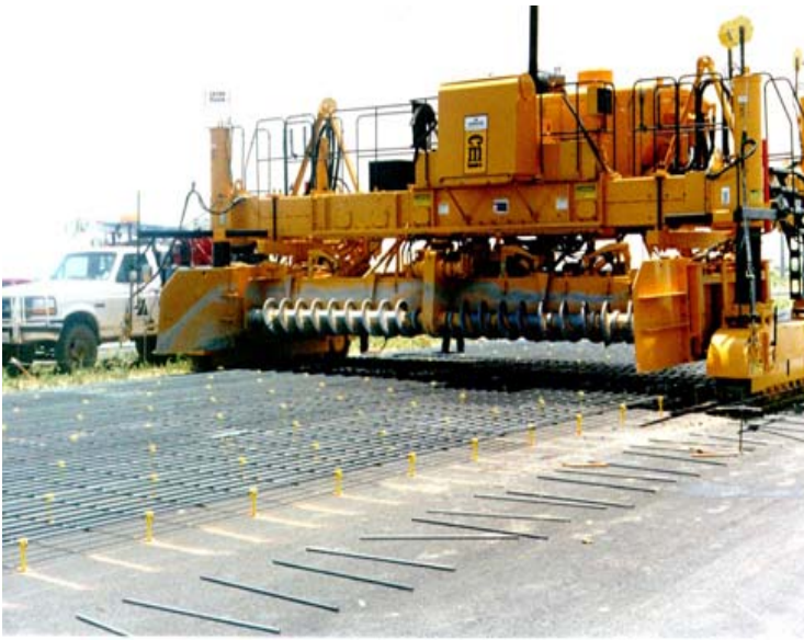
Figure 9-32. Slip-form paver with two augers (idle).
