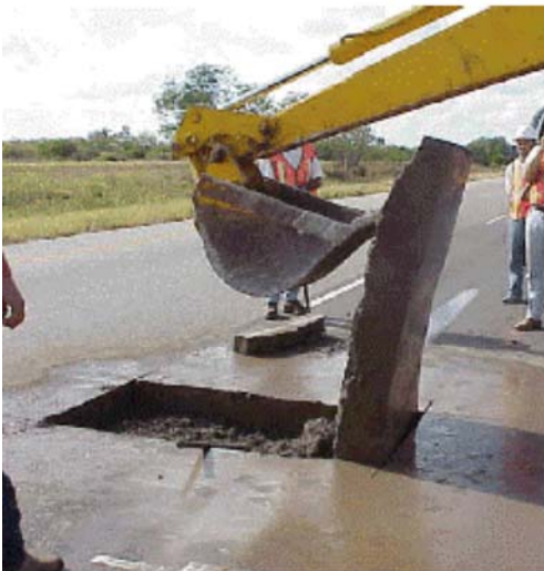
Figure 4-20. Flipping hot-mix asphalt (HMA) block out with backhoe.
