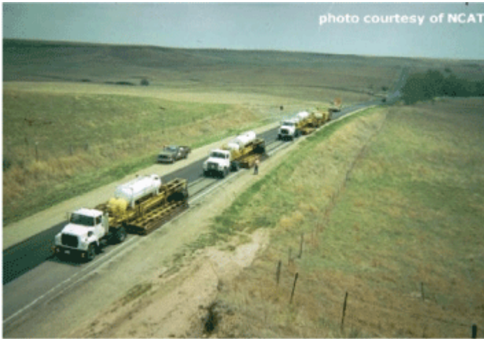
Figure 7-1. Hot In-place Recycling Train.
