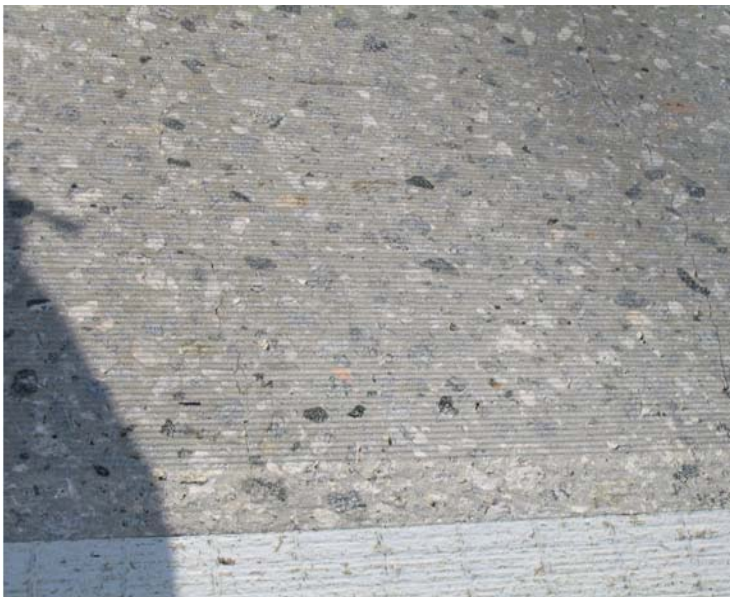
Figure 10-28. Close-up view of diamond ground surface.
