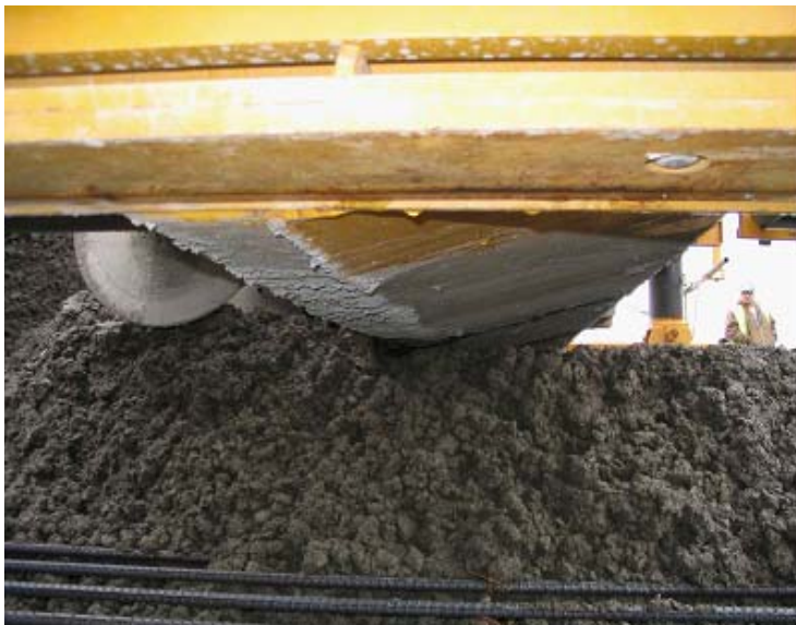
Figure 9-43. Auger and strike-off spreading the concrete.
