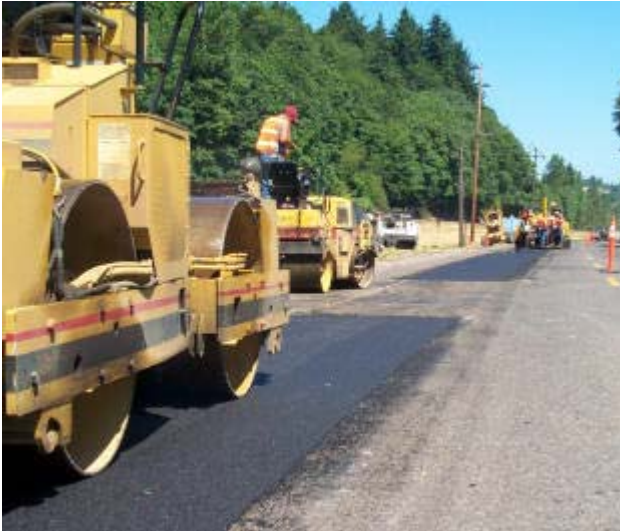
Figure 6-2. Repairing Failed Pavement Sections before Overlay.
