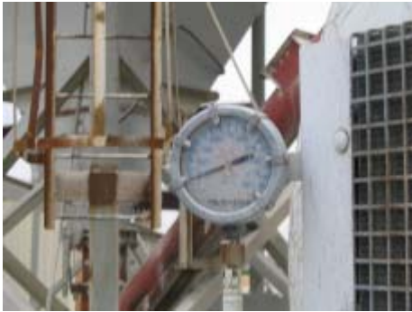
Figure 9-11. Slump meter mounted in the mixing truck.
