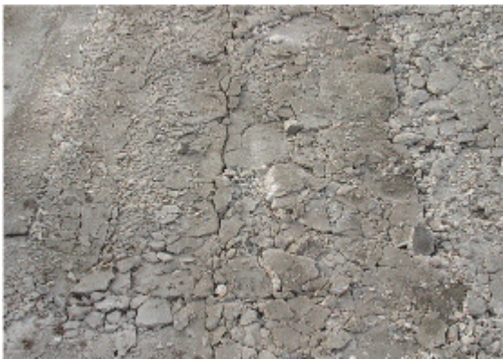
Figure 7-7. Rubblized pavement texture following resonant pavement breaking. © Copyright 2006 University of Washington
