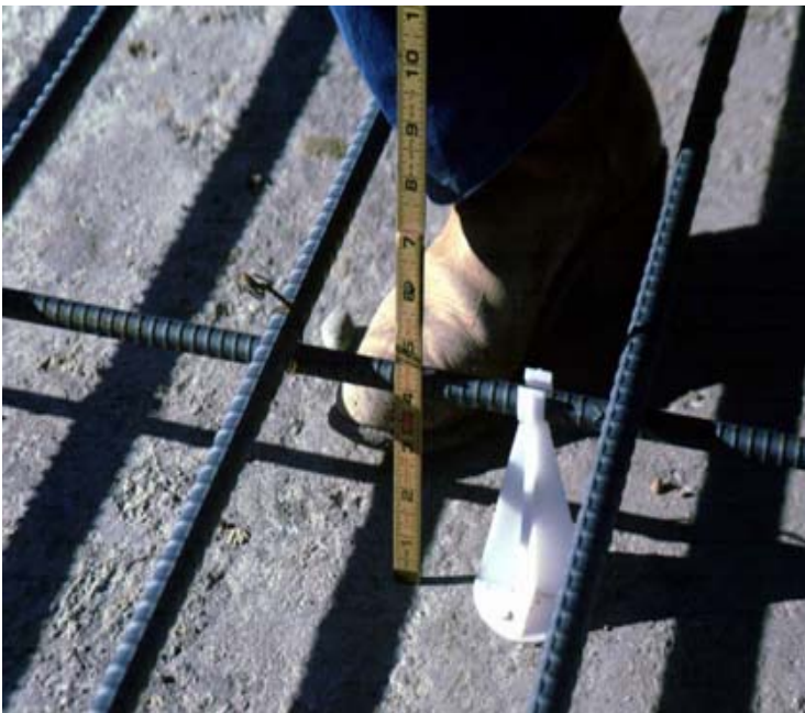
Figure 9-20. Checking steel location.
