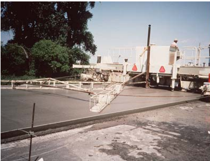
Figure 9-52. V-shaped drag float pulled by paver.
