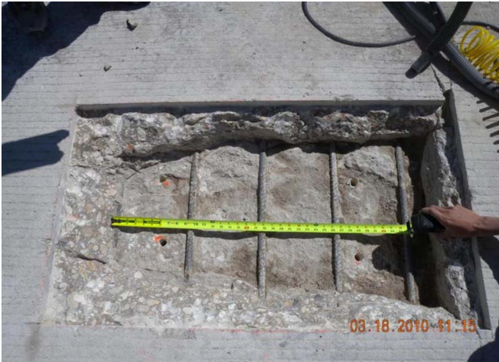
Figure 10-11. Clean repair surfaces.
