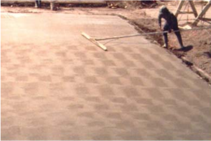
Figure 9-56. Straightedge finishing behind a longitudinal float.
