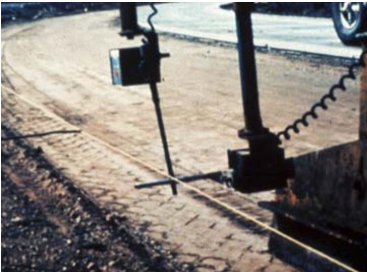
Figure 9-37. Horizontal and vertical sensors.
