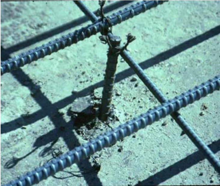
Figure 9-19. Pinning the mat.
