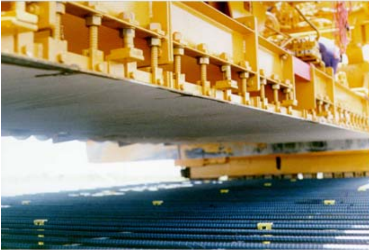
Figure 9-49. Looking up at a pan float on an idle paver.
