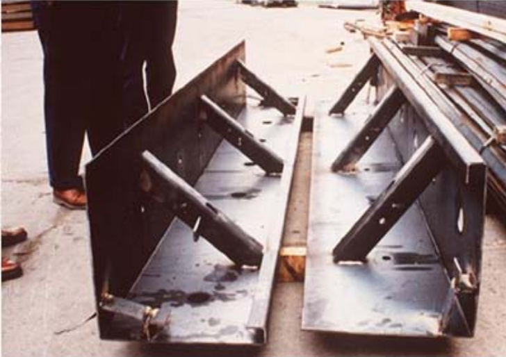
Figure 9-21. Forms ready for setting.
