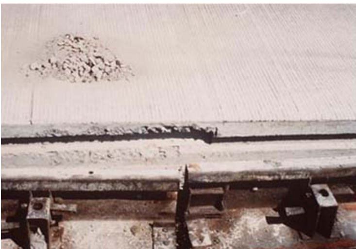
Figure 9-30. Removed side forms.
