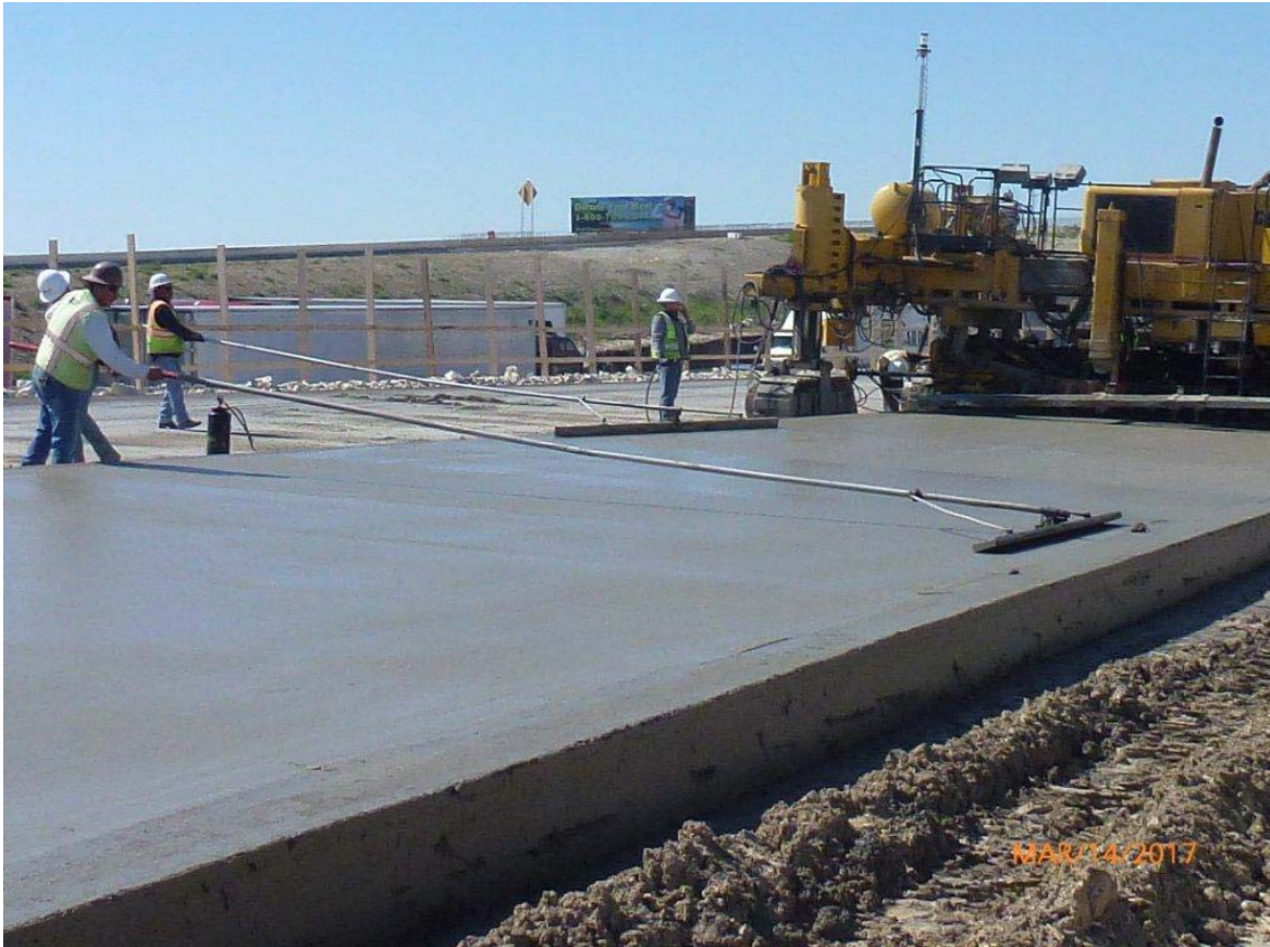
Figure 9-55. Straightedge finishing.
