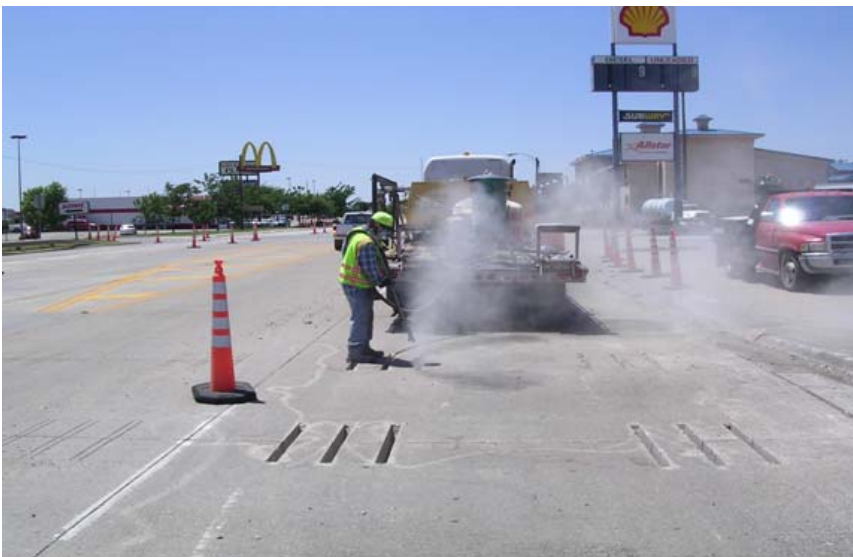
Figure 10-21. Sandblasting the slots.
