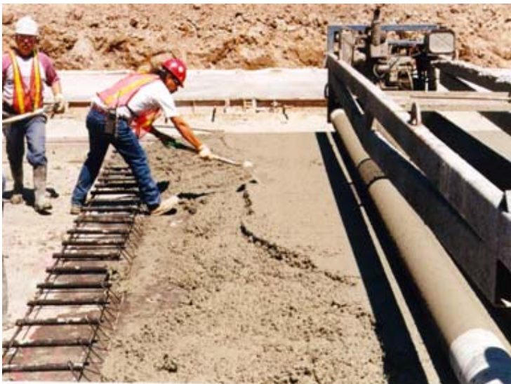
Figure 9-28. Knock down the ridge of mortar formed by the Clary screed.
