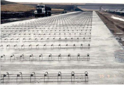
Figure 9-70. Dowel bars.
