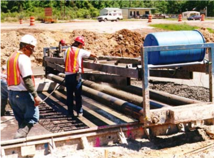
Figure 9-29. Cleaning screed between haul trucks.
