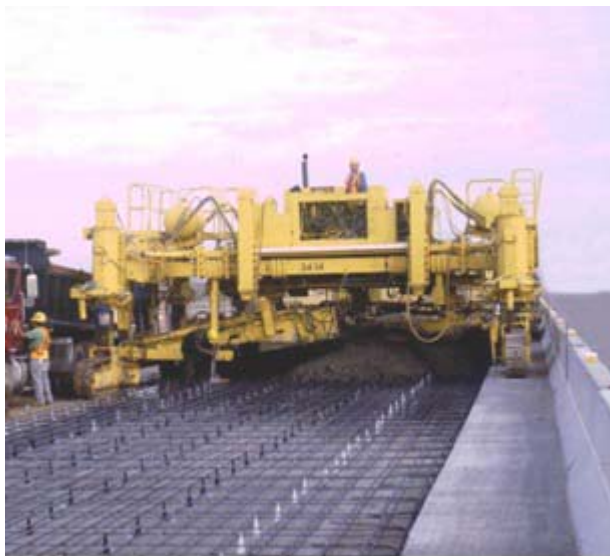
Figure 9-33. Paver machine on tracks.
