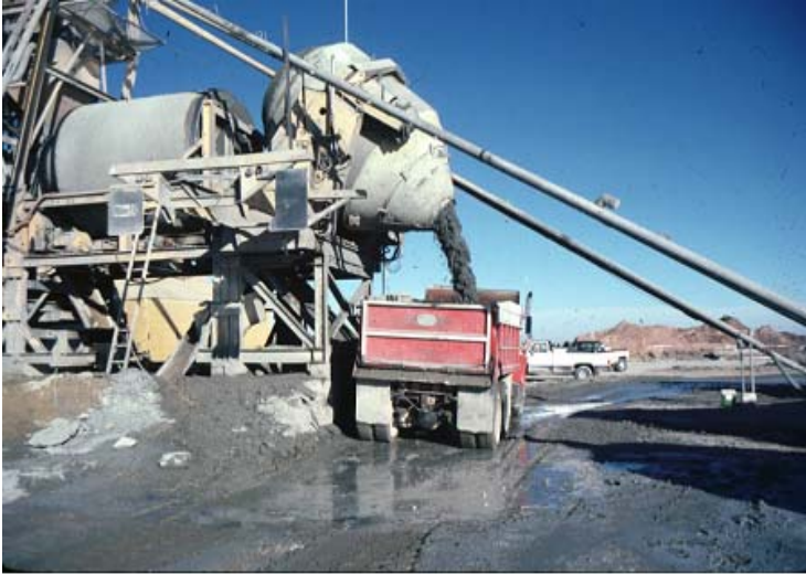
Figure 9-8. Discharging concrete into a dump truck.
