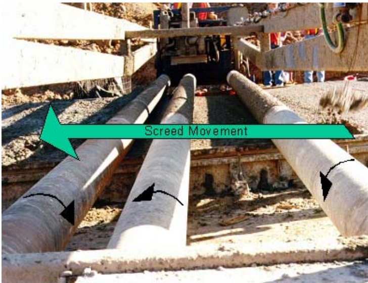
Figure 9-27. A Clary or roller screed.
