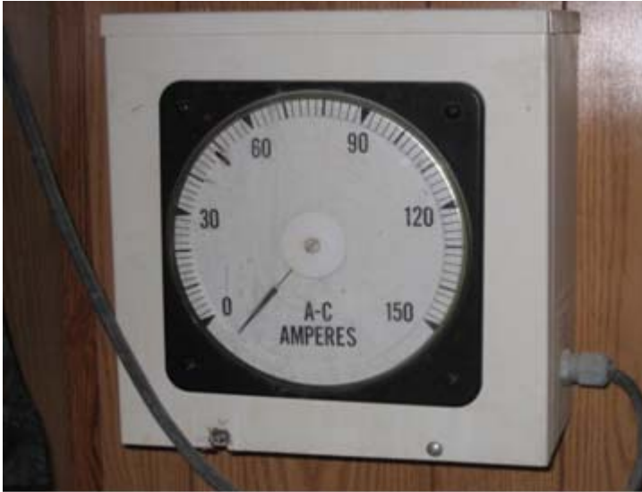
Figure 9-4. Amp meter for workability.
