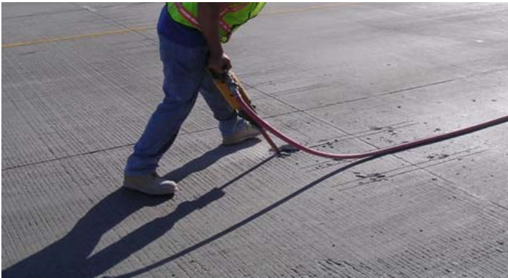
Figure 10-20. Removing concrete fins.
