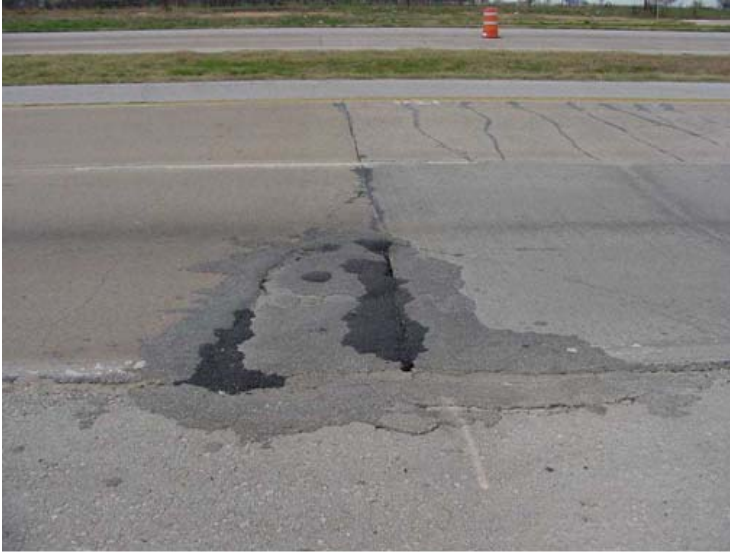
Figure 10-3. Full depth repair of punchouts in CRCP.
