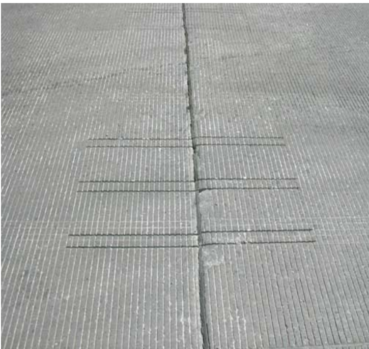
Figure 10-19. Cuts made for slots.
